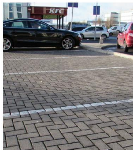
Permeable pavement (installed 2008) Finglas
